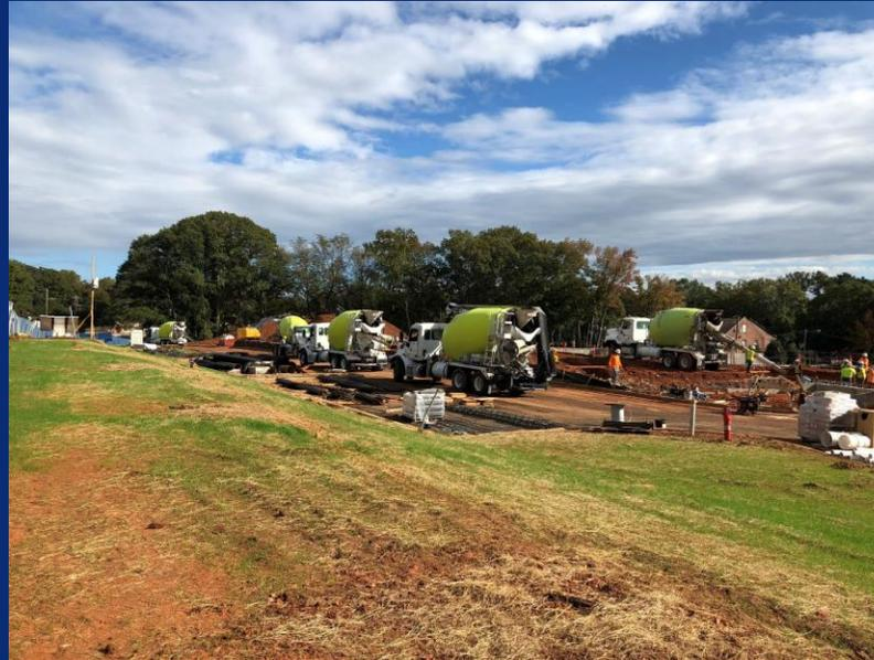
Concrete truck convoy on site for braced frame foundations
