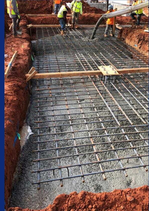
Braced frame foundation being poured
